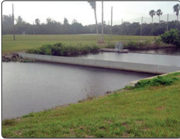
Diverters have quickly become an essential component of stormwater management and their applications have been used in a number of canals and other water flow systems. These diverters help the totality of a stormwater management system and are vital in combating the problems associated with runoff.
