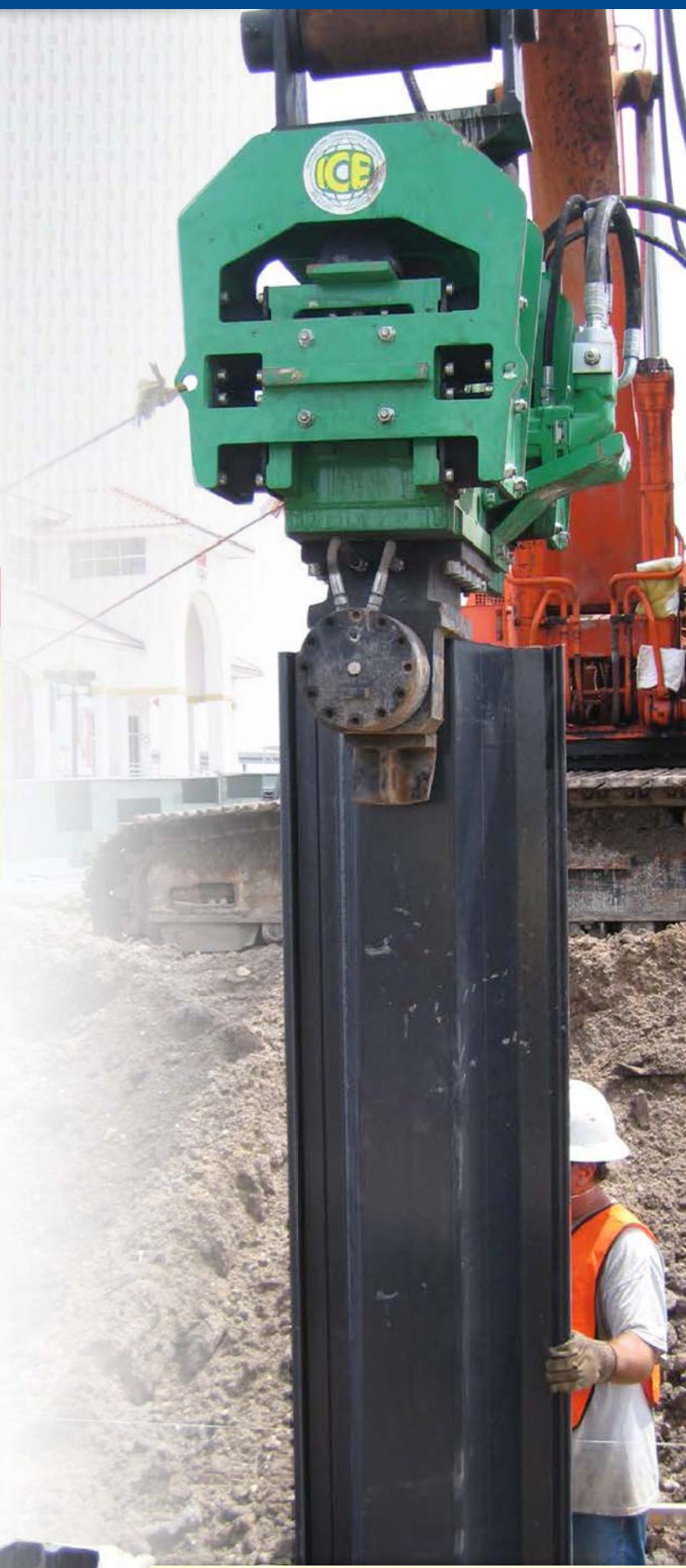
Vibratory Hammer Installation Example
