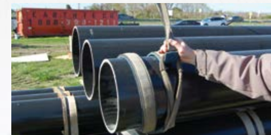
Lift-It® Sling Double Wrapped Around SUPERPILE®
