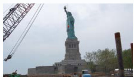
Liberty Island Installation Site
