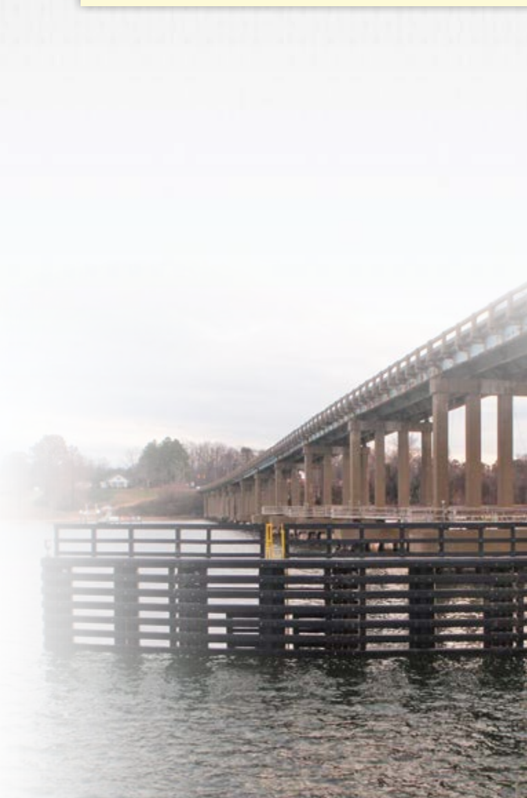
Fender Rehabilitation Route 3 Over Piankatank River, Virginia
